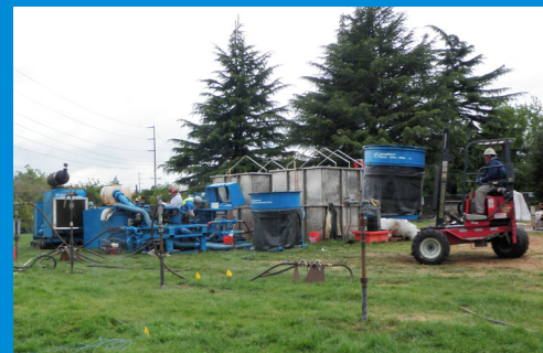
GeoSierra offers cutting-edge patented technology for installation of permeable reactive barriers (PRBs) placed via trenchless hydraulic fracturing methodology
