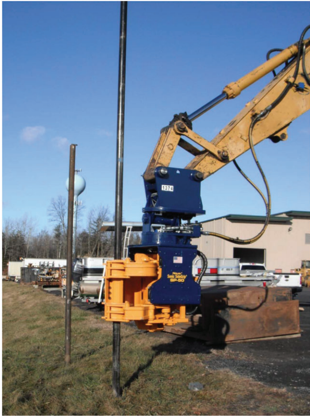
Figure 4. Direct-drive installation of ISTD heater casing.
